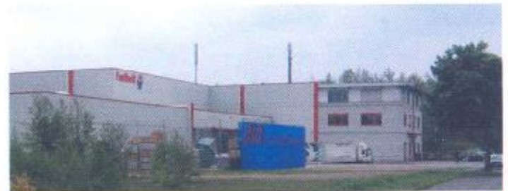
The Gronau warehouse now has major expansion potential
